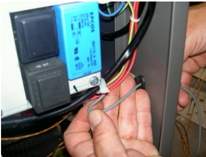
Fig. 1: Routing of cable through, rear panel
